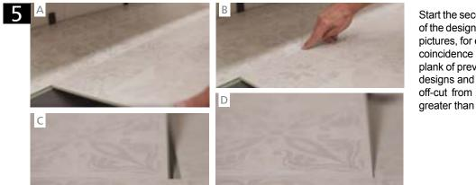
Start the second row, according the special features of the design choosen. In the design shown in these pictures, for example, plank has to be cut as per the coincidence of each tile bevels (around 50% of the plank of previous row). In the case of wood or stone designs and if their structure allows it, start with the off-cut from the previous row, provided its size is greater than 40 cm.
