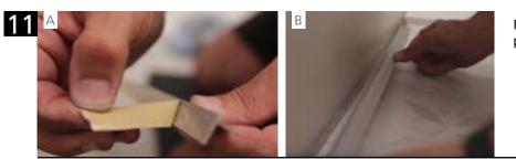
Remove the protective film . Place the skirting, pushing it till the complete fitting.
