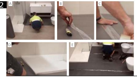
When laying Faus laminate flooring over any subfloor, a foam underlay with a moisture/vapor barrier must always be installed first ("underlay" FAUS ).
