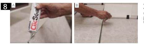
Generally there is no need to use it, but in areas with large and continuous water spills, it is highly recommended to apply our Click Seal Floor joint sealant. Apply to the flooring tongue before laying the plank. Remove any surplus.
