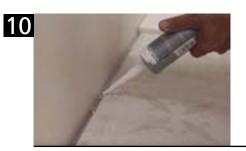
After measuring and cutting the profiles, it is time to apply flexible silicone in all the area between floor-wall and planks to fill in the expansion gap.
