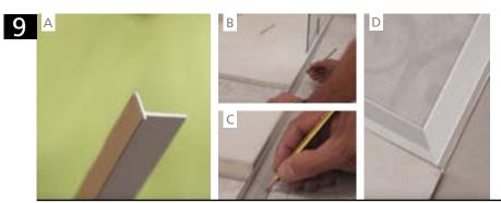
Prepare the aluminium skirting. Place the adhesive side on the wall (do not remove the protective film up to step 11), the bottom side of the profile must be laid on the expansion gap. Put first the aluminium profile and mark the cuts. It is very important to make mitre cuts.
