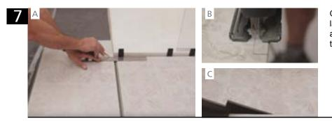
On areas where full length planks can not be laid, measure and trace a guide line with a pencil along the surface. Take in mind always to leave the expansion gap.
