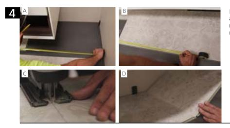
Insert the short end of the next plank in angle and snap it to the first one. Continue along the row. Cut the last board of the row to fit it in (it is necessary to use a saw for wood).
