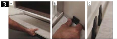
Start in the left-hand corner and lay the first plank, the tongue side of the board (the less machined edge) facing the wall and place plastic spacers between the wall and the plank. We suggest to trim the tongue outgoing to avoid any problems with the expansion gaps. Leave 10 - 12 mm expansion gaps all around the walls and other fixed elements.
